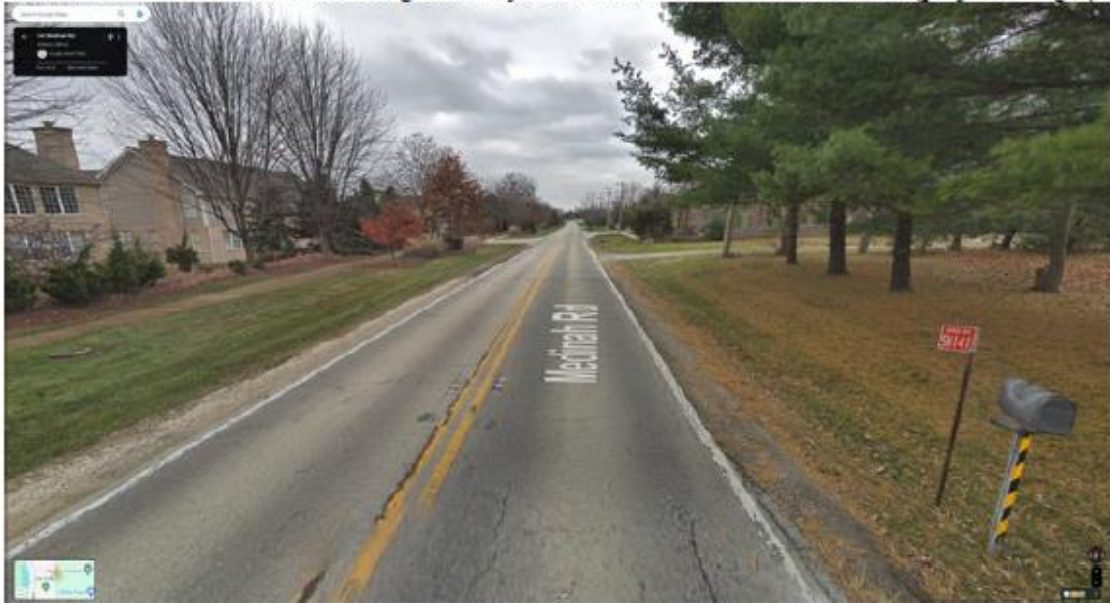
Medinah Road further north looking mid-way between Erie Circle & Nicola Ct. (project to right)
