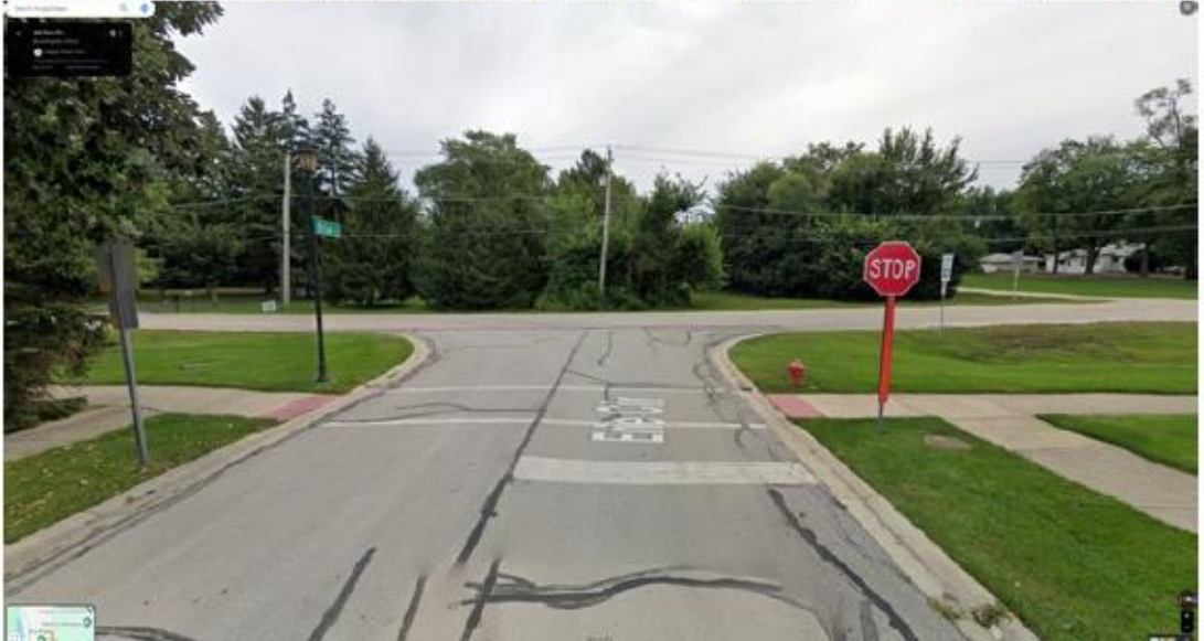
Erie Court Intersection with Medinah Rd. looking east (towards proposed south project entrance)
