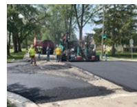
Crews pave over the final stretch of the Country Club Highlands project.
