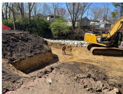
V3 construction crew work to excavate the area for installation of a concrete spillway, which will be the entry point for stormwater into the facility from St. Joseph Creek.
