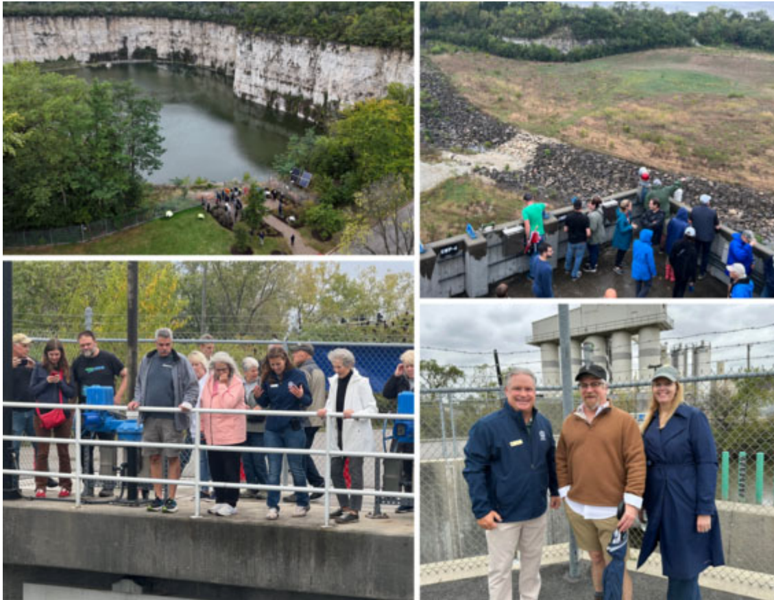
Visitors enjoyed rare views of the inner workings of the Elmhurst Quarry Flood Control facility from three vantage points. Bottom Right: SWM Chair Jim Zay kicked the tours off with Elmhurst Aldermen Karen Sienko and Guido Nardini..
