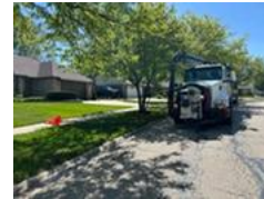
SWM equipment and personnel deployed to Peters Court in Downers Grove Township to assist with flushing out a blocked sewer.
