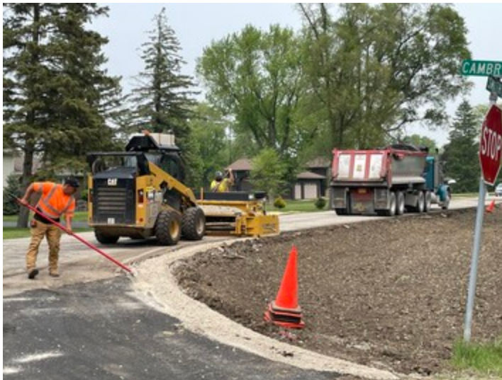
Crews place stone shoulder along Smith Road, one of the final tasks needed to consider the project substantially complete.
