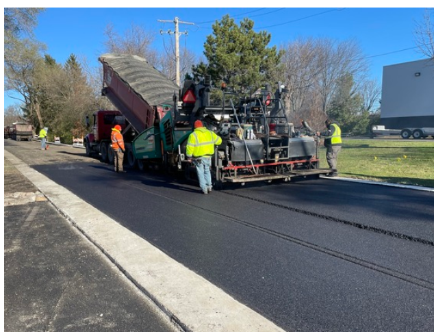
Work crews lay down fresh asphalt over the new storm sewer system installed in unincorporated Lombard as part of the Luther High Ridge Flood Relief project.
