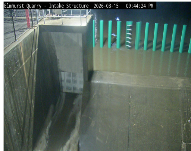
A camera feed from the Elmhurst Quarry Intake Structure shows water flowing in at 9:44 PM on Sunday, March 15.
