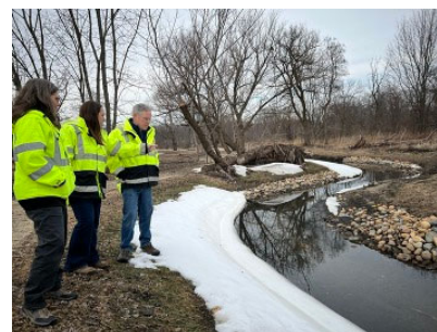
SWM Committee Chair Jim Zay joined staff for a tour of the Winfield Creek Streambank Stabilization Project site, where installed native plants will soon bloom.
