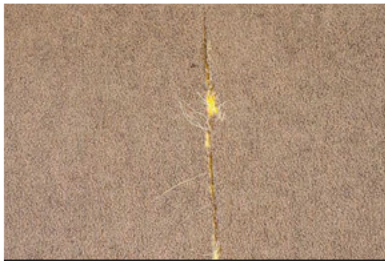
Ripped and fraying carpet at the seam in second floor
