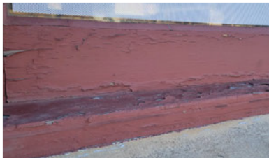
Peeling window frame. Frames up on the west side are worse.
