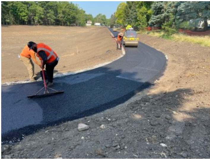
V3 Construction crew install an asphalt pedestrian path around the Main Street Flood Storage Facility.
