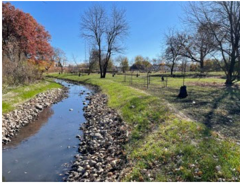
A freshly restored portion of Winfield Creek, featuring a stabilizing rock toe along the bank and new trees planted in the adjacent wetland area.
