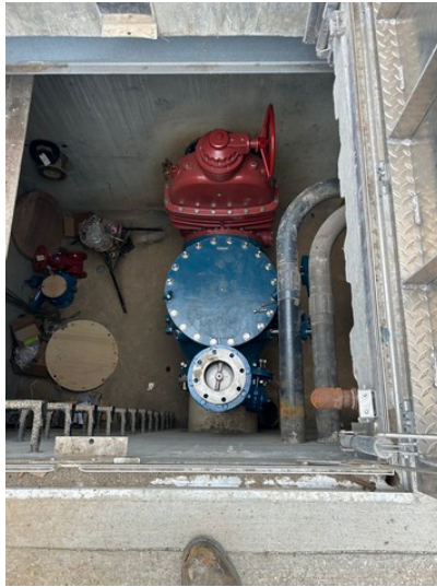
A panel opens at the Quarry to show the newly installed check valves and piping, which are critical to efficient operation.
