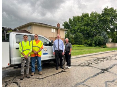
State Senator John Curran and SWM Chair Jim Zay pose in front of the completed drainage project, along with two members of SWM's field crew who worked on the project.
